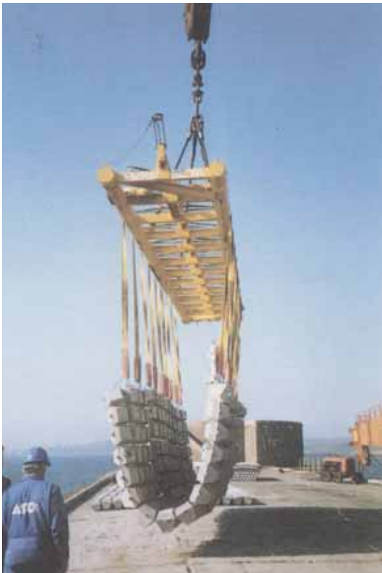
Figure 3.22: Concrete Mattress being Lifted by a Lifting Frame
