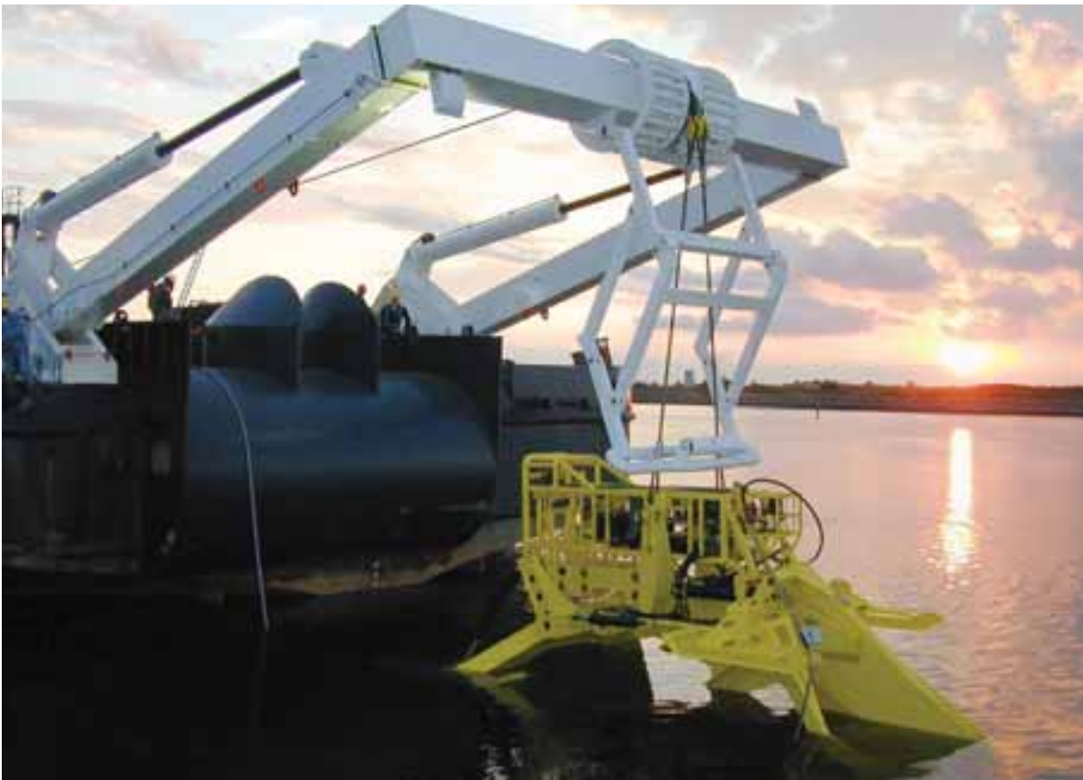
Figure 3.12: Cable Plough Launch and Recovery from a Host Vessel
